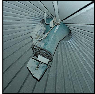
Photo 3 -- Close-up view of grain spreader in the bin.
